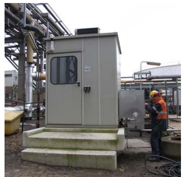
ODS project with walk in shelter and fast sample loop
