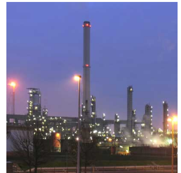
Hazardous zone in the petrochemical Industry.
