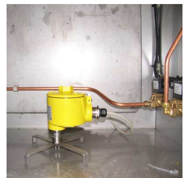
An FCI level switch shuts off the sample pump in case of a leakage
