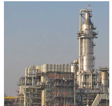
Short sample lines implements the use of Ex analyser houses
