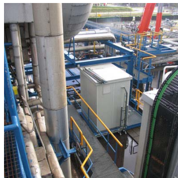
ODS analyser shelter for a return condensate project
