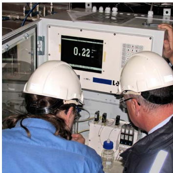
Commissioning and start up
