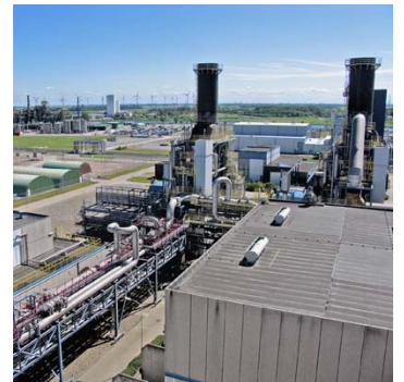
Power plant met co-generators
