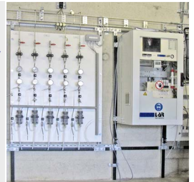
ODS multi-stream TOC-analyser for return condensate
