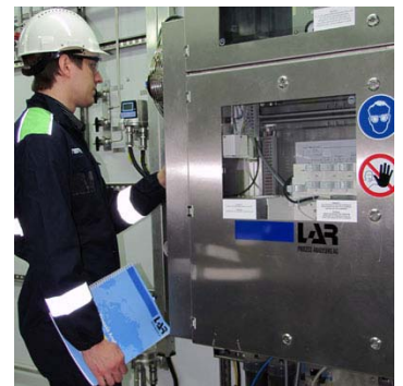
Inspection of an ATEX zone 1 Quick-TOC-analyser
