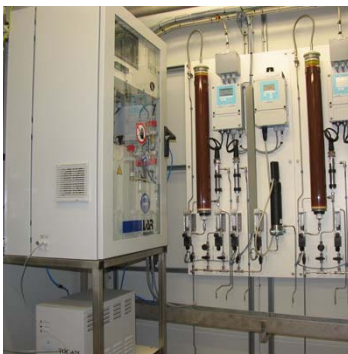
The TOC-analyser mounted in a walk-in analyzer shelter
