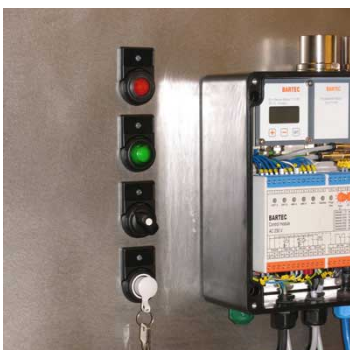
Control switches EEx-p cabinet
