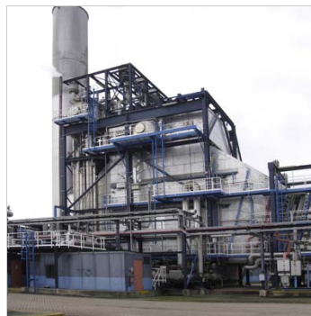
Co-generator. ODS installed three return condensate TC-analysers
