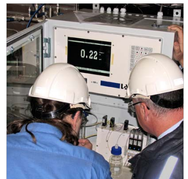
Service engineers inspect the Quick-TOC-condensate analyser
