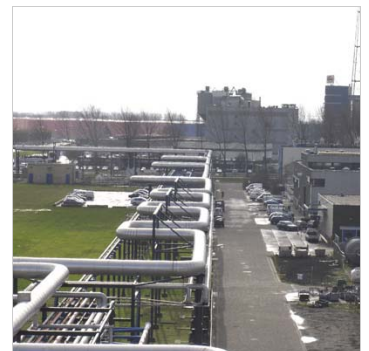
Transport pipes with Return Condensate
