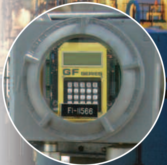
Transmitter/Readout in optional explosion proof aluminum enclosure
